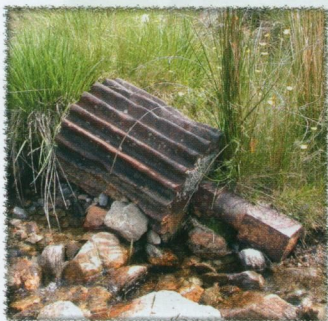
Rusting gear from the waterwheel at Corranree
